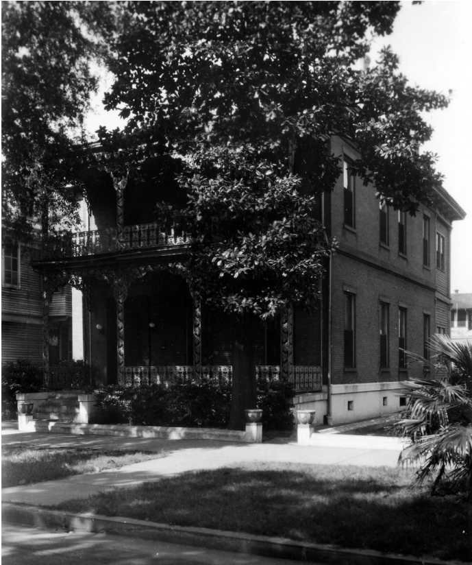
Peter Burke occupied this house at the north west corner of Government and Scott streets, along with his wife, Maggie, and her parents, Owen and Margaret Finnegan. In the mid-twenties it became Higgins and Courtney, a funeral home and was eventually lost for a gas station. A fried chicken franchise occupies the corner today.
