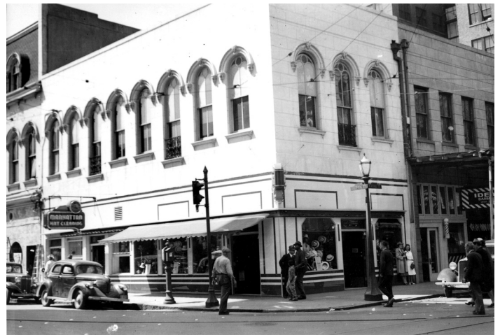
By the 1930's the Burke Building had lost its third floor to a fire and the popularity of cigars had plunged. Here it houses a men's hat store. In recent years a cast iron gallery has been put back onto the structure.
